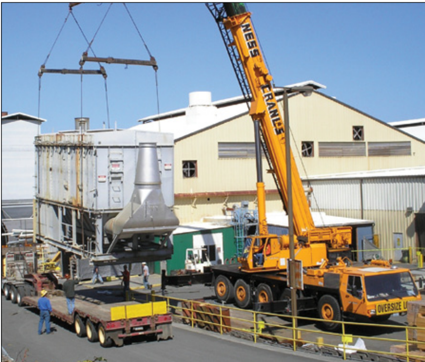
Dust Collection System Replacement improves workspace air quality while cutting Compressed Air consumption by 47% in glass manufacturing facility.
