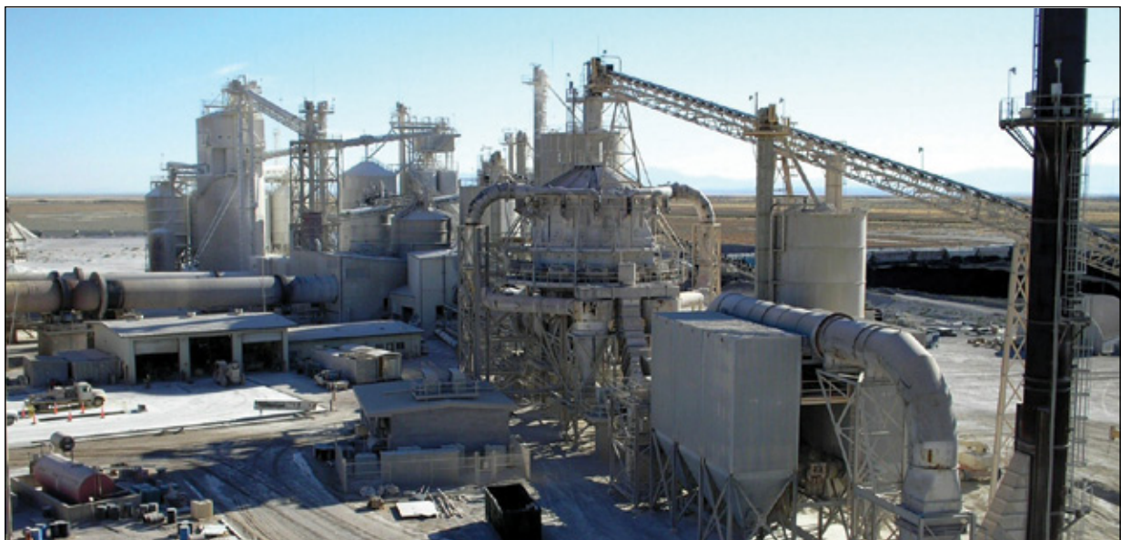
Energy efficiency improvements reduce power consumption of kiln by more than 30% at remote mining operation.
