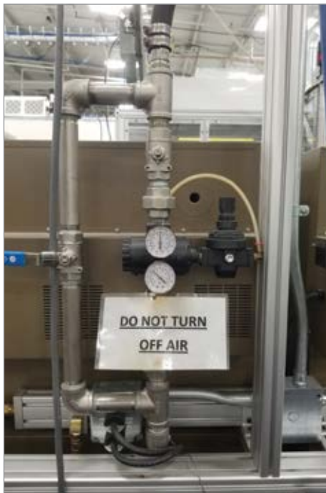
Many flow controllers are now used in lieu of PSI regulators.
