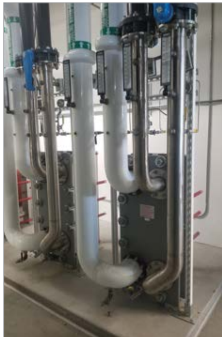
Heat of compression is recovered and effectively used to heat water.
