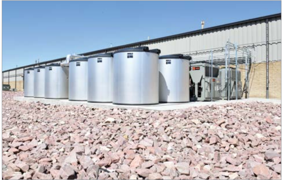
A cool thermal energy storage system uses stored ice or chilled water as a medium for deploying energy. (Image courtesy of Trane.) There is hot and cold thermal energy storage. Hot TES would include the water heater in your home. This article focuses on cool thermal energy storage including chilled water storage and ice storage.
