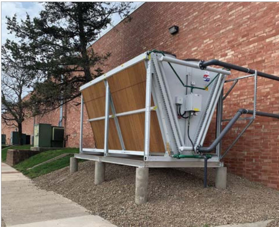
An adiabatic chiller helped saved 10 million gallons of water annually at a Berry Global plant.
