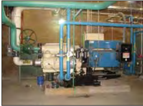
Ingersoll Rand Centac® 800 hp 3 stage Oil-Free Centrifugal Compressor
