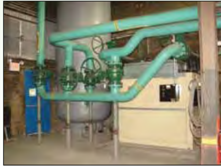
Ingersoll Rand Variable Capacity Refrigerated Dryer and Receiver
