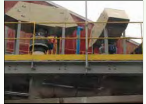
Ingersoll Rand Centac® Dual Inlet Filter Assemblies
