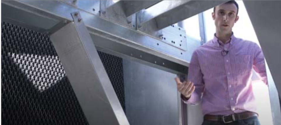
A crossflow cooling tower's large plenum area allows easy maintenance.
