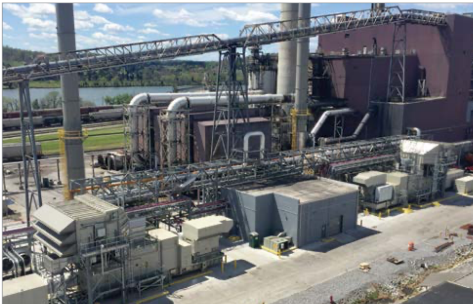
Tate & Lyle operates the only two U.S. EPA Energy Star accredited corn wet mills in the U.S. including its facility in Loudon, Tennessee.
