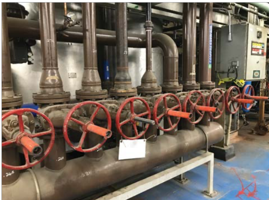
Compressed air average pressure, flow and dew point is measured and monitored.
