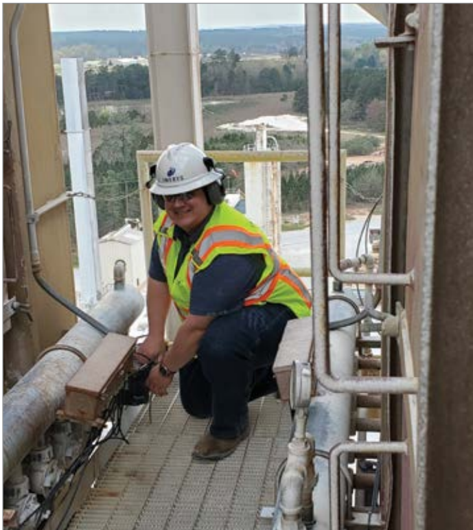
Robin Davis of Imerys Performance Mineral Americas installs a technically advanced pulse valve that has proven to improve dust collector performance and reduce compressed air consumption.
