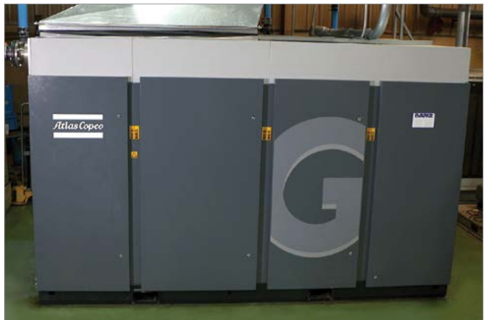
An oil-injected, 300-hp Atlas Copco GA 250 VSD rotary screw air compressor automatically matches compressed air supply to demand at Douglas Autotech’s Hopkinsville facility, resulting in substantial energy savings.
