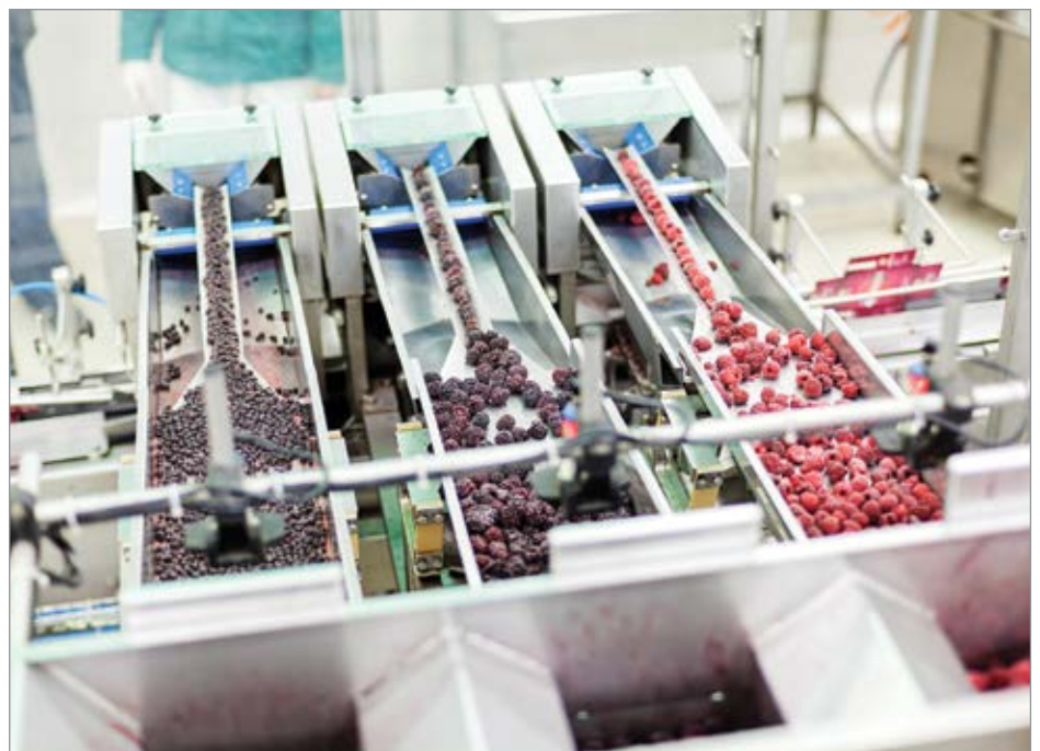
Carefully planned designs and preventive maintenance are key to managing risks associated with compressed air systems.
