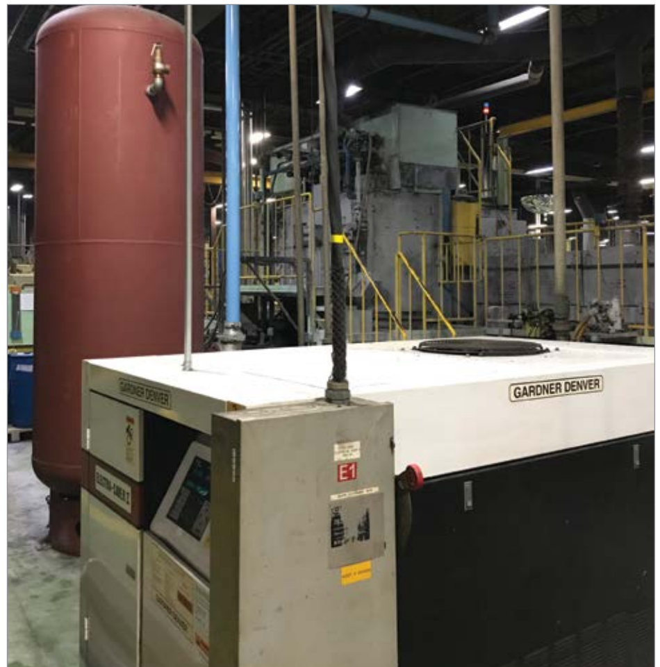
As part of its compressed air system upgrade at its Midway plant, SumiRiko Tennessee installed a 1,000-gallon receiver tank to provide additional compressed air storage for its wet blasting operation.
