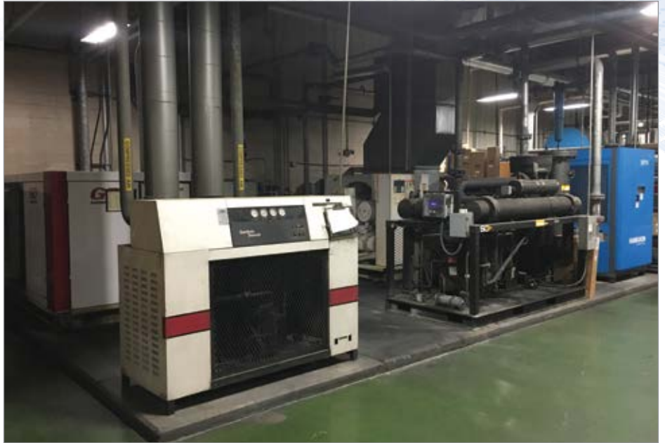
Shown is one of five rotary screw air compressors used to supply compressed air to power production areas at SumiRiko Tennessee's Midway plant.
