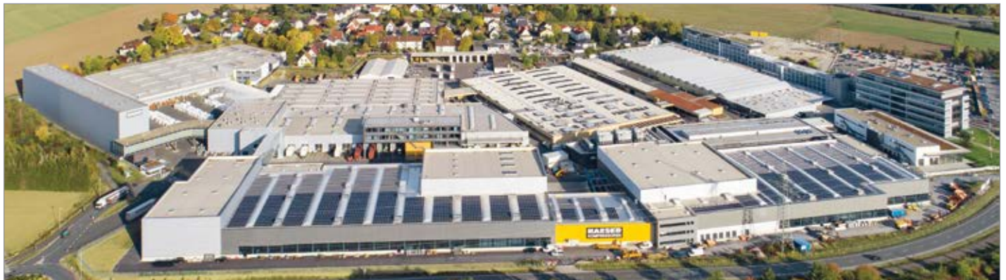
Aerial View of Kaeser Kompressoren in Coburg, Germany
