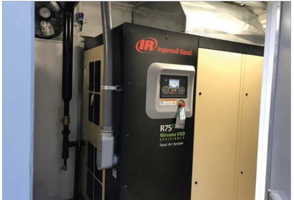
The compact air compressors, with integrated dryer/filter packages, are all housed in the same cabinet, allowing three air compressors to be placed inside the sea container with room to spare.
