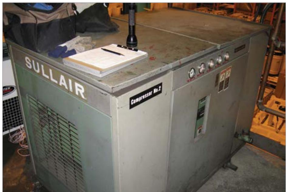
Shown is a 25 hp fixed speed unit rated to deliver 100 cfm.
