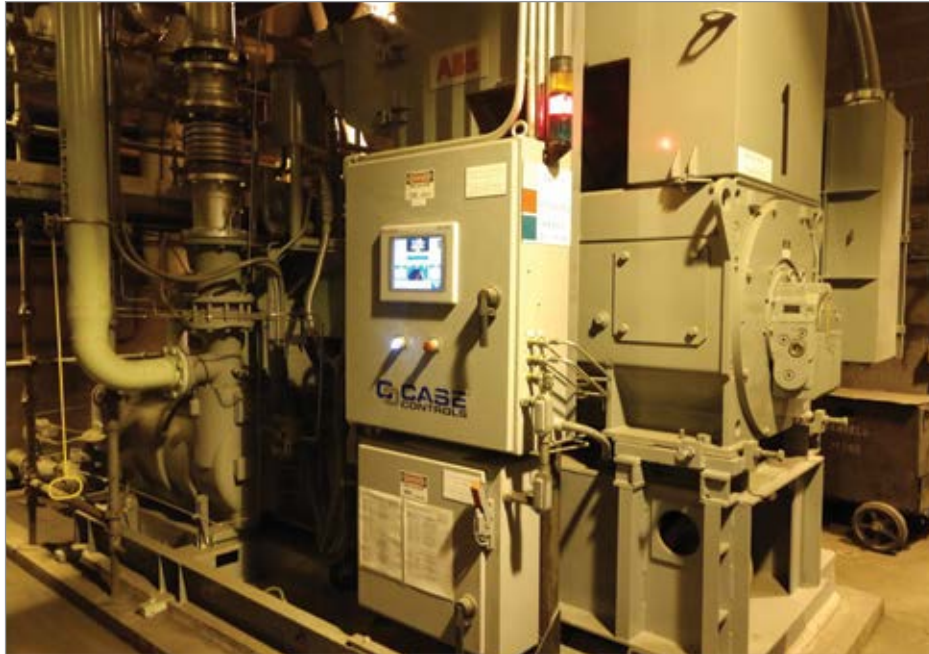
Shown is an AirLogix controller on a centrifugal air compressor. The machine is one of three units networked with an AirMaster master controller.
