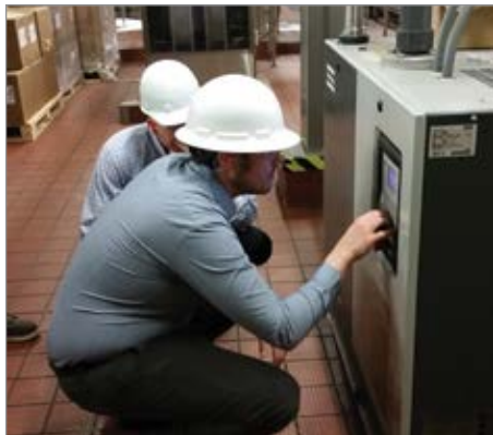
Atlas Copco GHS VSD+ rotary screw vacuum pump at Widmer Brothers Brewery.
