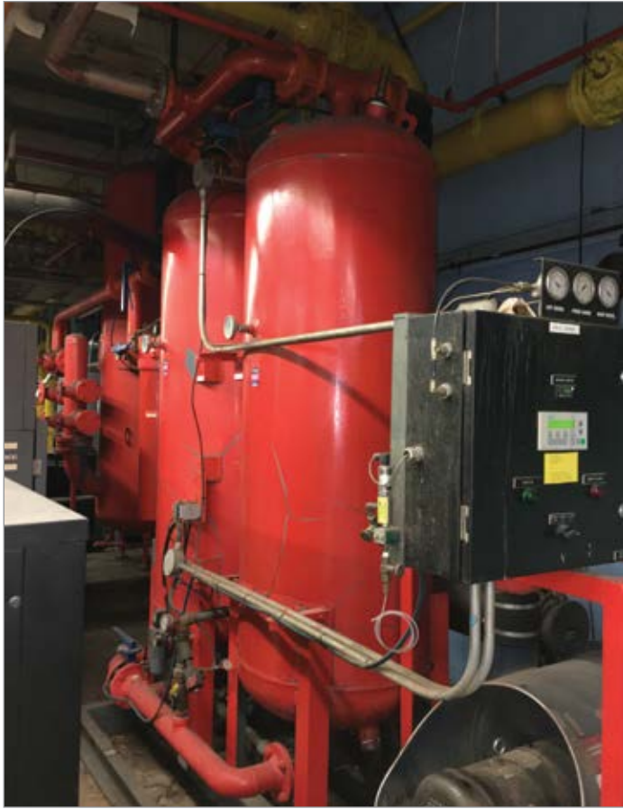
Figure 3: The heated blower style dryer maintains a -40 °F pressure dewpoint.
