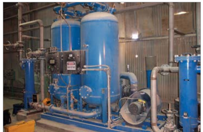
A heated blower style desiccant dryer takes up considerable floor space, but the use of ambient air for purge saves energy. (The surrounding dust hints at problems to come.)
