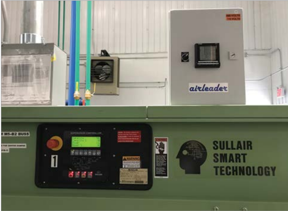
An Airleader control module installed on an air compressor at North American Lighting.
