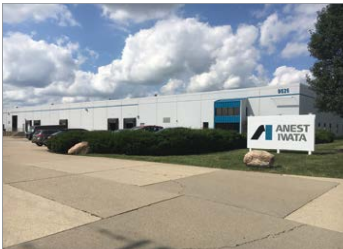
Anest IWATA Air Engineering's new 53,000 square foot facility.
