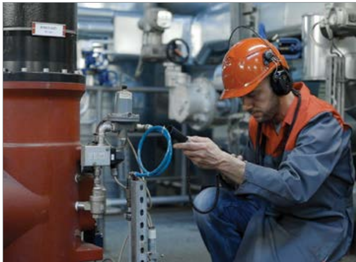
Leaks are broadband phenomena as the LeakExpert app on the SONAPHONE easily demonstrates
