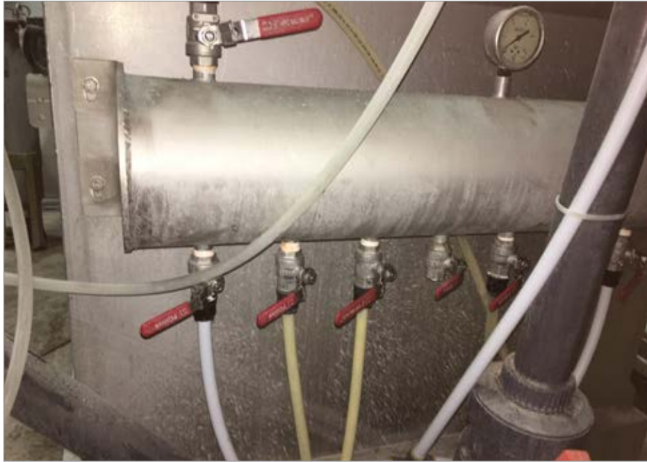
Figure 5: Air agitation of a sewage treatment vessel is a potentially inappropriate end use.
