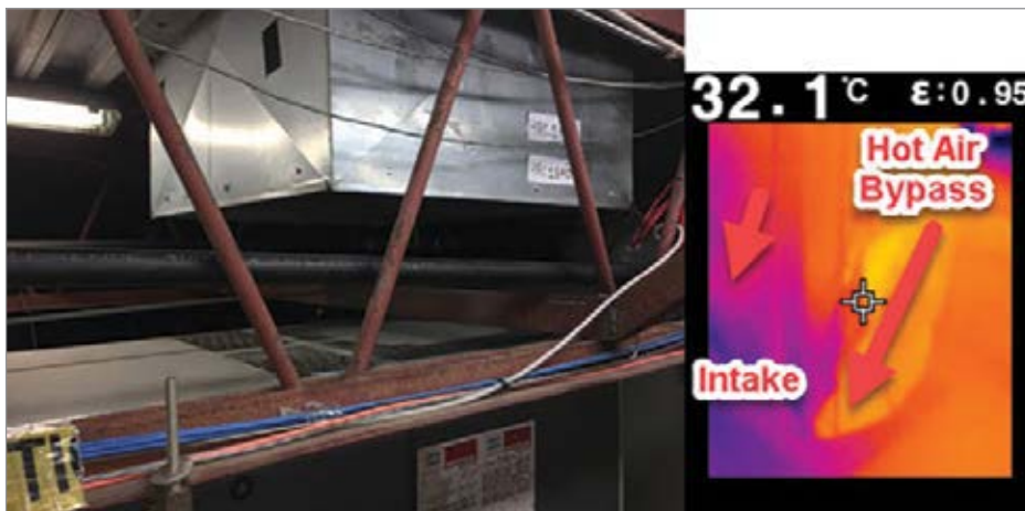
Figure 6: The lack of continuous ducting (left) allows hot air to spill into the cooling intake of both the compressors (thermograph right) and dryers causing overheating. This becomes obvious when looked at with a thermal camera.
