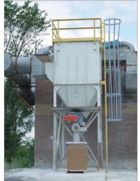
The LST System is a typical pulse jet dust collector for waste product.
