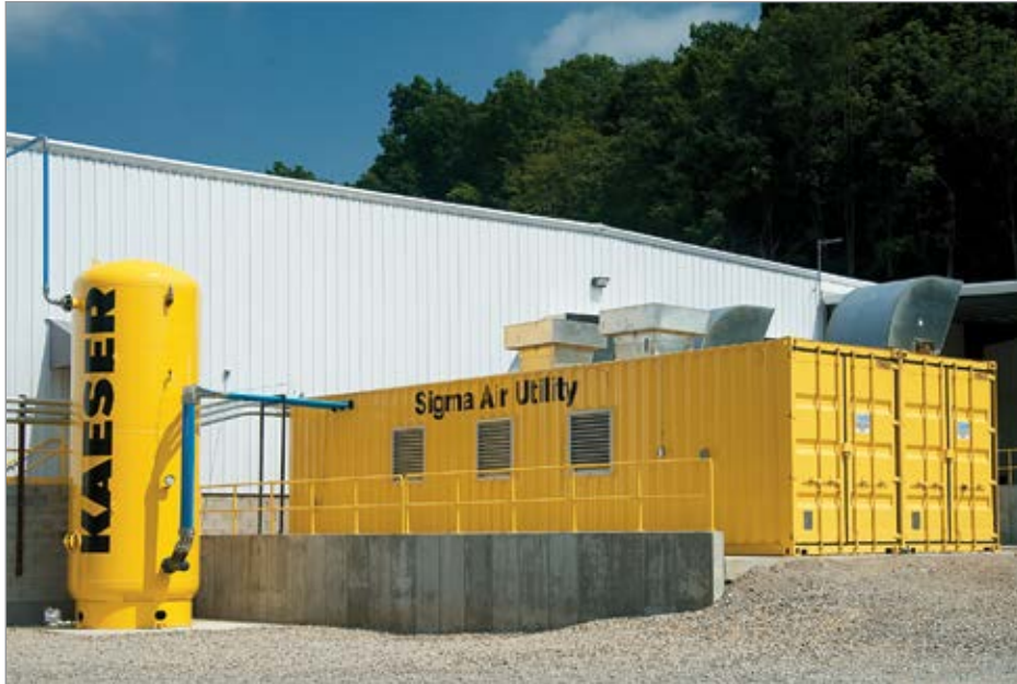
Planning, installing and operating the Sigma Air Utility system is Kaeser's responsibility, allowing users to save on the investment and maintenance costs of a compressed air system.
