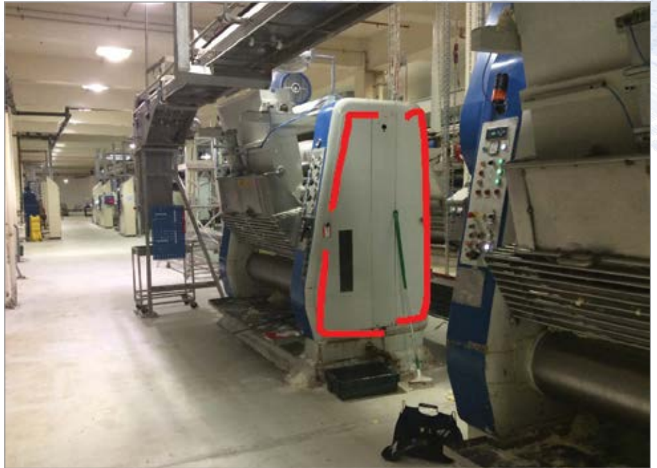
One machine can have several leaks.
