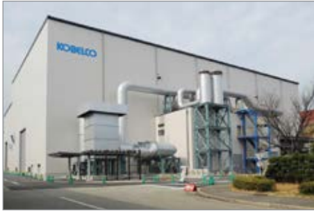
Kobe Steel's 40 MW compressor test facility is designed to meet the growing need for large-capacity compressors in the world market.
