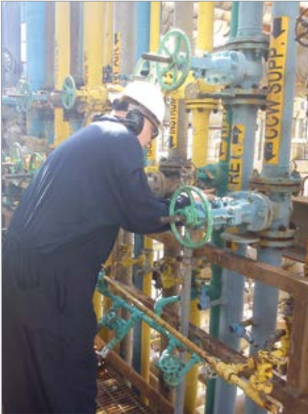
PCE measures leak loss by orifice size, plume length, and line pressure. We can find leaks in areas that would be unnoticed and undetected by the human ear.
