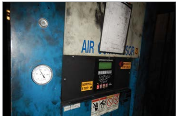
Figure 6: To better control this compressor of another brand, IAC integrated a Sullair microprocessor and Airleader took direct control of the poppet valves to control part loading of this unit.
