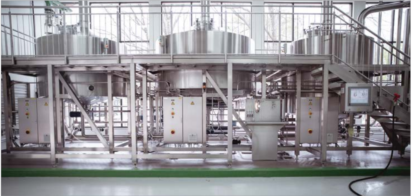
Brewery equipment using nitrogen generated onsite from the compressed air system.
