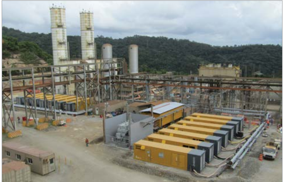
Atlas Copco ZH6000 and ZH9000 units are self-contained, 100 percent oil-free, three-stage centrifugal air compressors that fit completely within a standard 40-foot shipping container. Electrically powered, the units have zero risk of exhaust contamination that can be a problem with diesel units.
