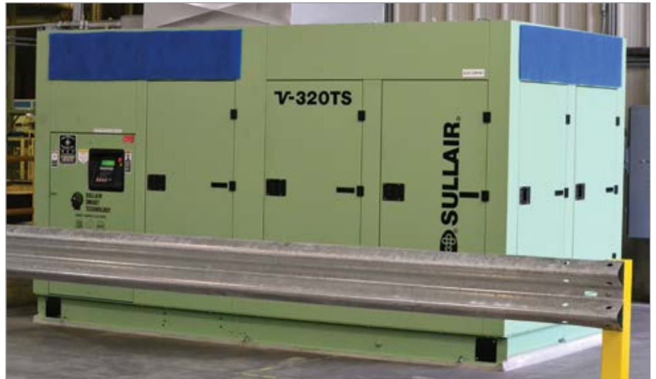
A $46,000 energy rebate helped finance the installation of a new Sullair V320-TS-250H two-stage tandem air compressor using two sets of rotors for full-load and part-load efficiency.
