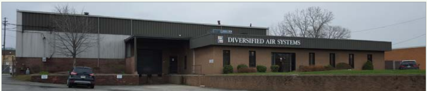
Diversified Air Systems, Inc. provides engineered compressed air solutions to Northern Ohio, Western Pennsylvania, Southern Michigan and the Pan Handle of West Virginia.
