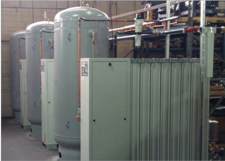
Figure 5: Peak Industrial i-Flow nitrogen generators are modular, and a system can use multiple units working in parallel.
