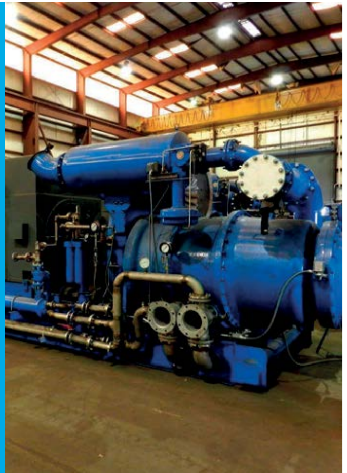
Figure 3: Internal view of the dual nitrogen generation system designed by Titus Air Systems
