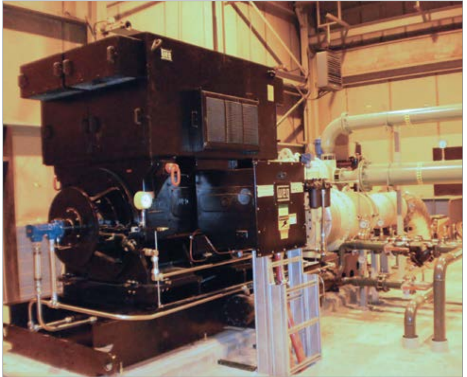
Figure 2: Replacing the old Turbo 5 with two new compressors has saved a significant repair bill, and has made the system more efficient.
