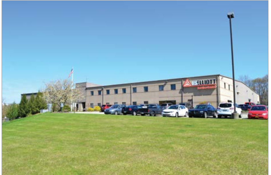
FS-Elliott's new service center in Export, PA
