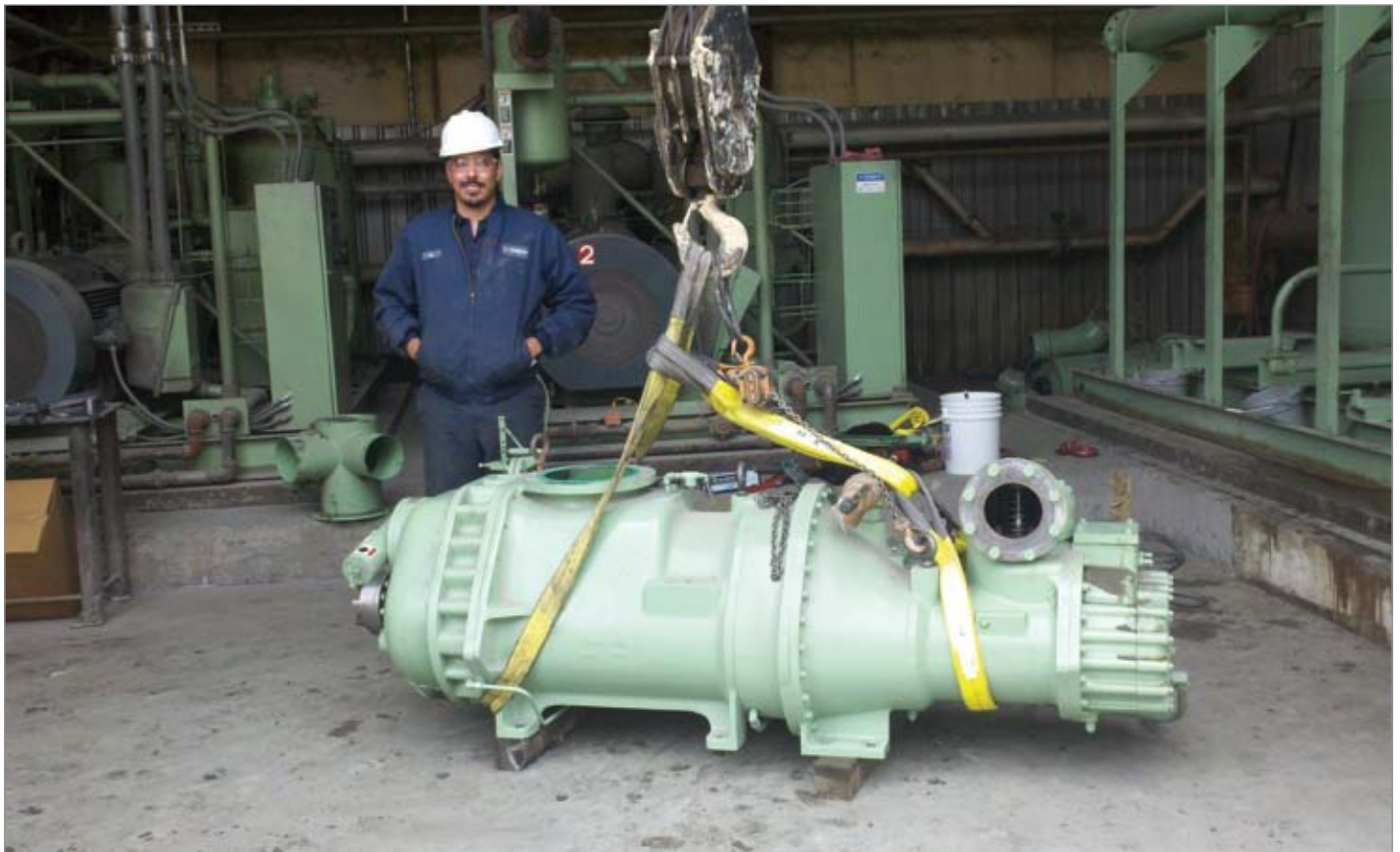
Northwest Pump & Equipment services all types of rotating equipment.
