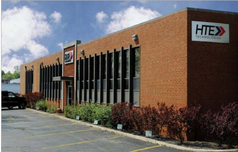
HTE Technologies is headquartered in St. Louis with a 6,500 ft 2 branch in Decatur, Illinois.
