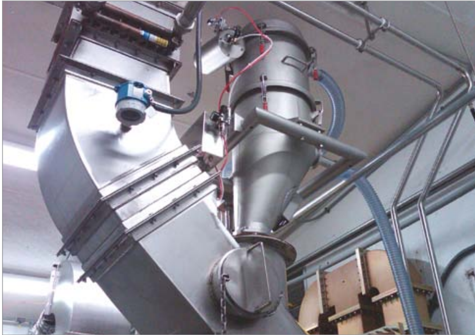
Nutriom uses two VAC-U-MAX pneumatic conveyors with a mixer — one system breaks the powder up and puts it into the mixer and the other pulls it out of the mixer.
