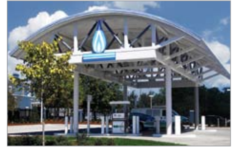
Public access NGV fast-fill refueling station.
