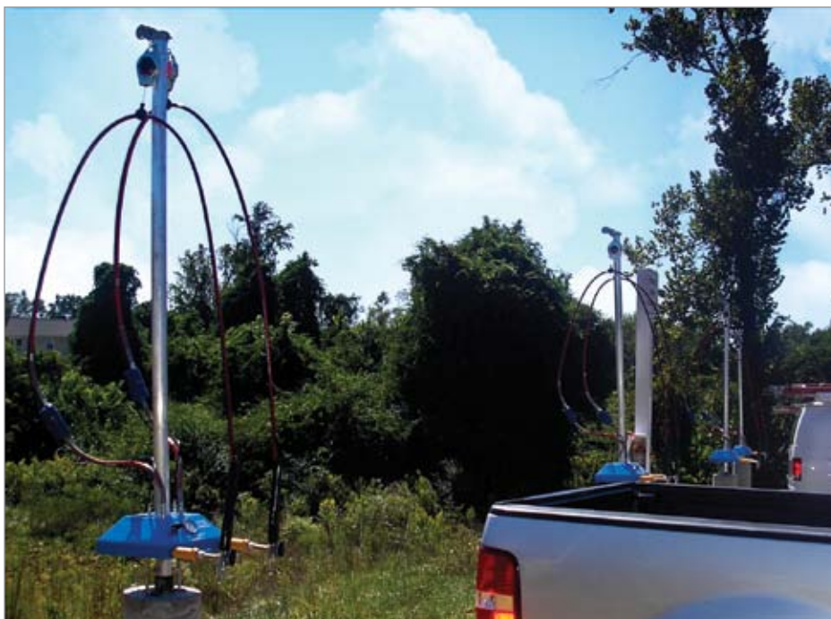
Twin-hose fill-posts for overnight refueling of a gas utilities' NGV service fleet.
