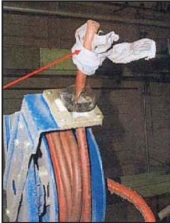
Figure 2. Check average size of leaks
