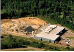
Aerial photo of NEWPRO particleboard plant, Smithers, B.C.
