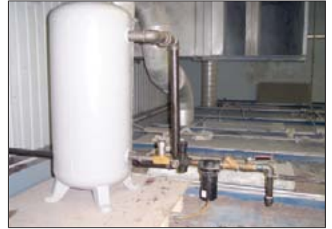
This metered recovery system enhances bag house pulses.
