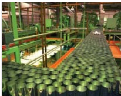
Leaks reduce compressed air pressure and increase spoilage costs in high-speed applications like can manufacturing.
