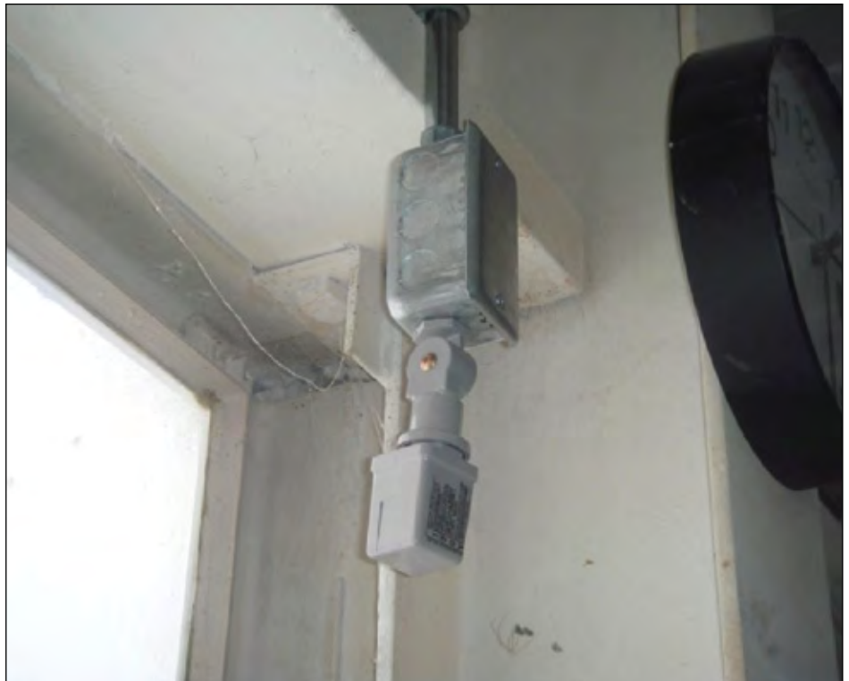
#6 A simple light sensor can shut down lights when the sun is shining
