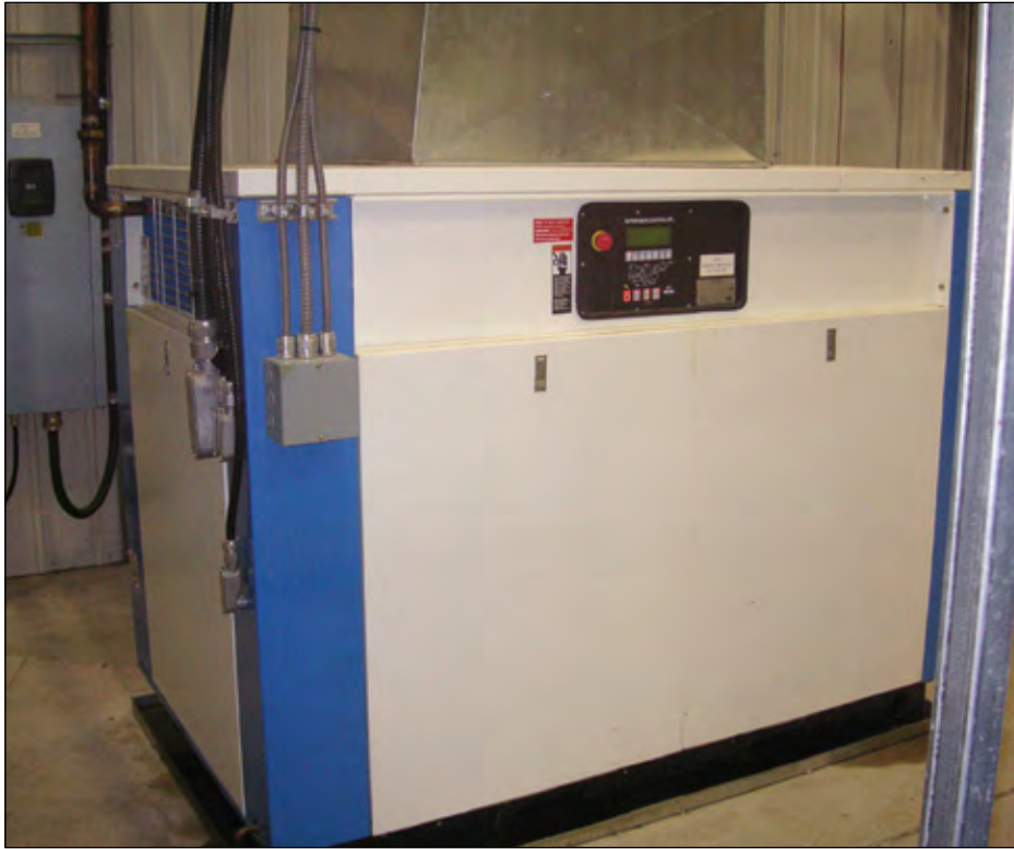
Variable Speed Compressor efficiently matches the nitrogen generator demand
