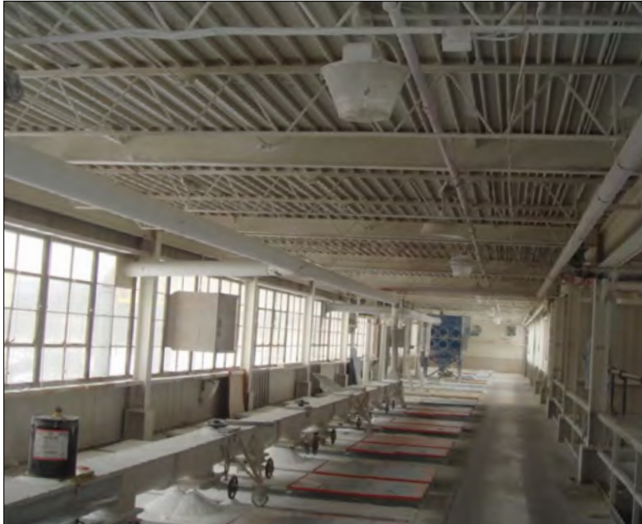
#7 These lights are turned off by sensors when the sunlight is available.
