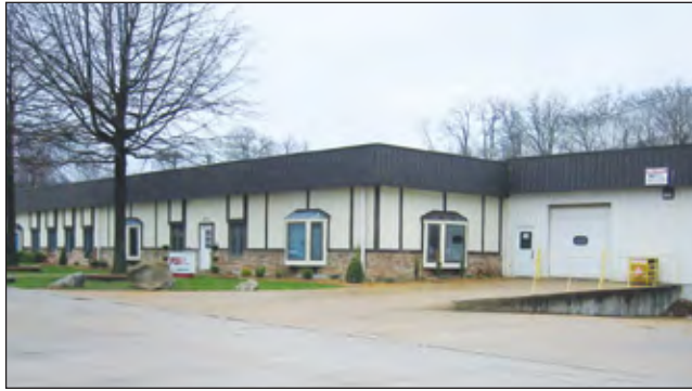
Power Supply Industries Headquarters in Fenton, Missouri
