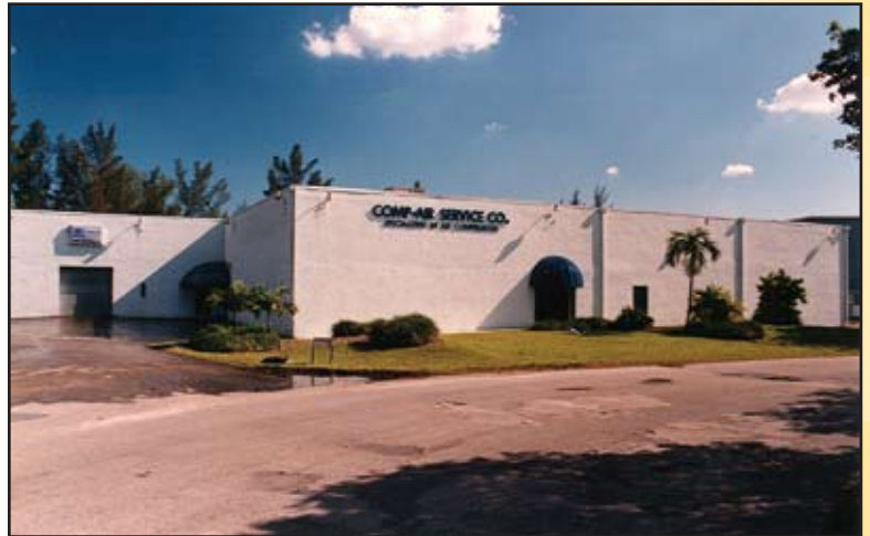
Comp-Air Service Company Headquarters in Miami, Florida
