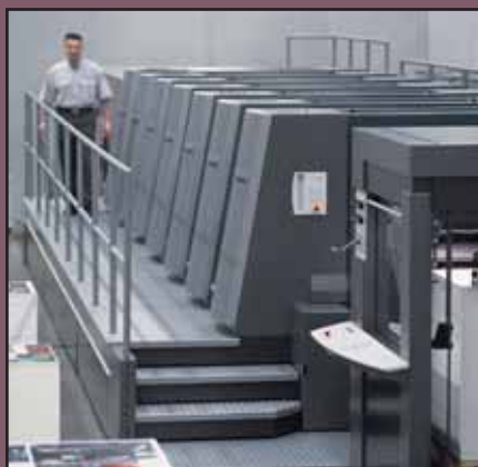
Vacuum systems in commercial printing offer just as many energy-efficiency opportunities as does compressed air (Illustration: Heidelberg Druckmaschinen AG).
