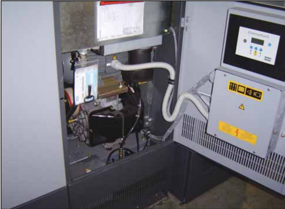
Heidelberg Scrollstar® System featuring an Atlas Copco scroll compressor with an integrated refrigerated dryer.
