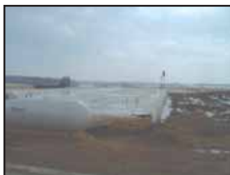
Step 3: Digester at Dairy Farm
