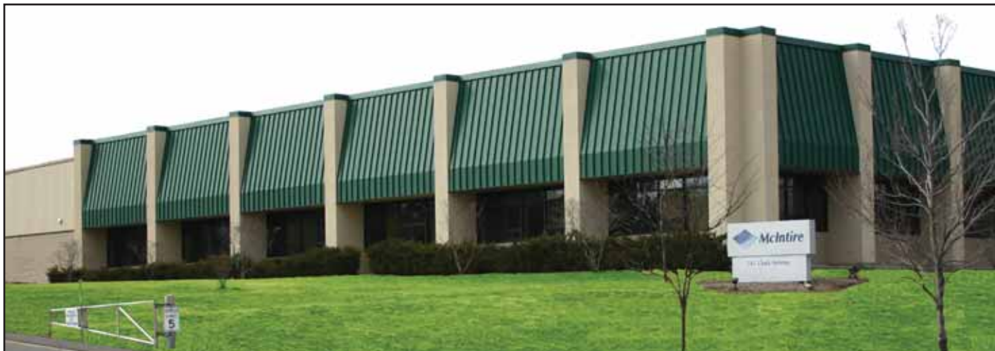
McIntire's new home was built in 1999 and is dedicated to the manufacture of compressed air dryers.
