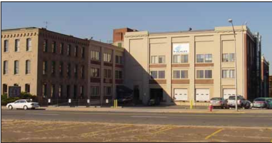
Scales Connecticut Service Facility
