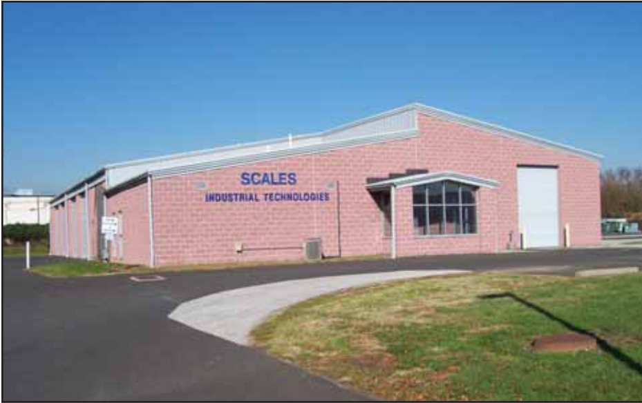
Scales Philadelphia Service Facility
